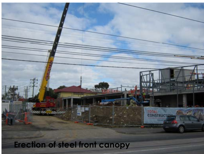
Canopy steel framing
