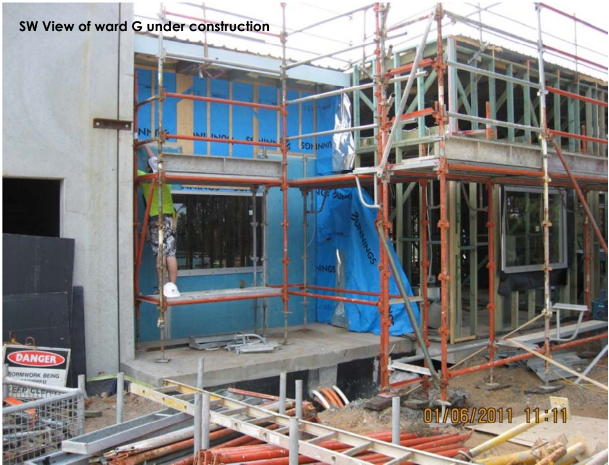
Precast panel installation
